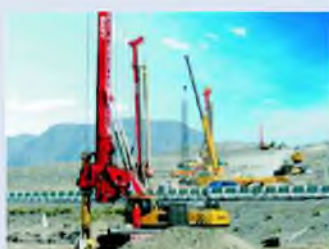
Rotary drilling rig
